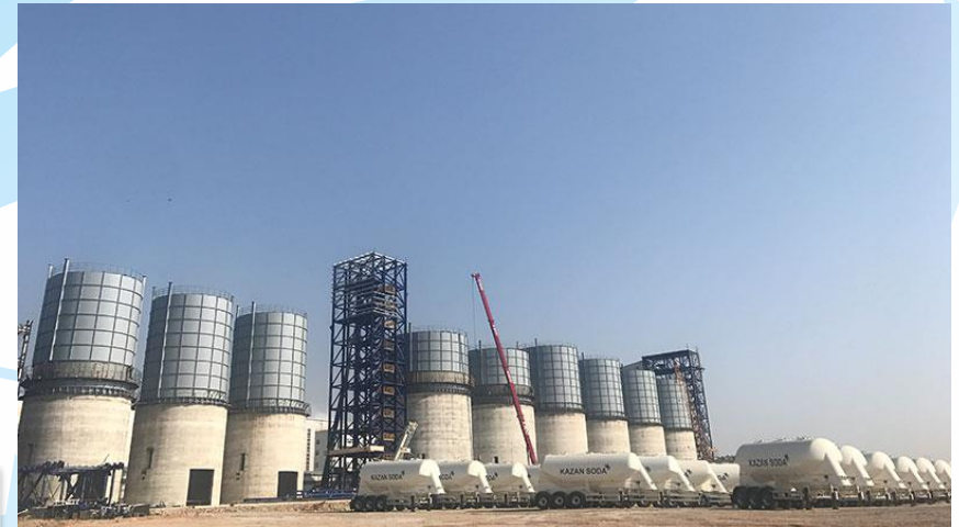
Turkey's largest capacity cogeneration facilities with 380 MWe and 400 tons of steam production Kazan Soda Facility (Ankara)
